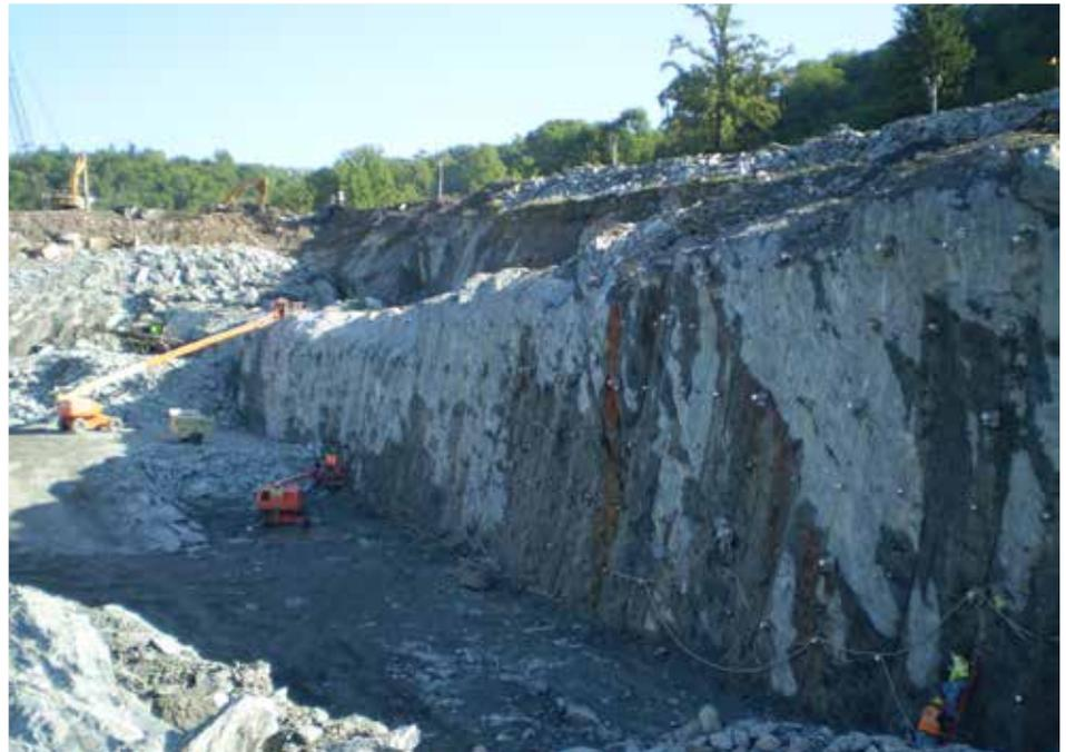
extensions, and tailrace to carry the water. Clearing each of the individual areas required extensive blasting through hard bedrock, as well as a support system to stabilize the slope and prevent future failures as large volumes of water flow down the Susquehanna through the power facility.
